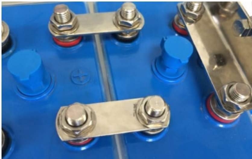
Fig.9. Fitting the interconnecting plates.
